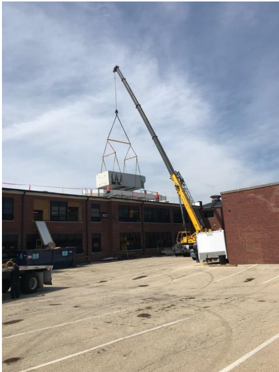
RTU Crane Lift
