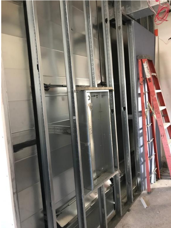
Duct Chase Framing
