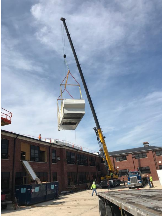
RTU Crane Lift
